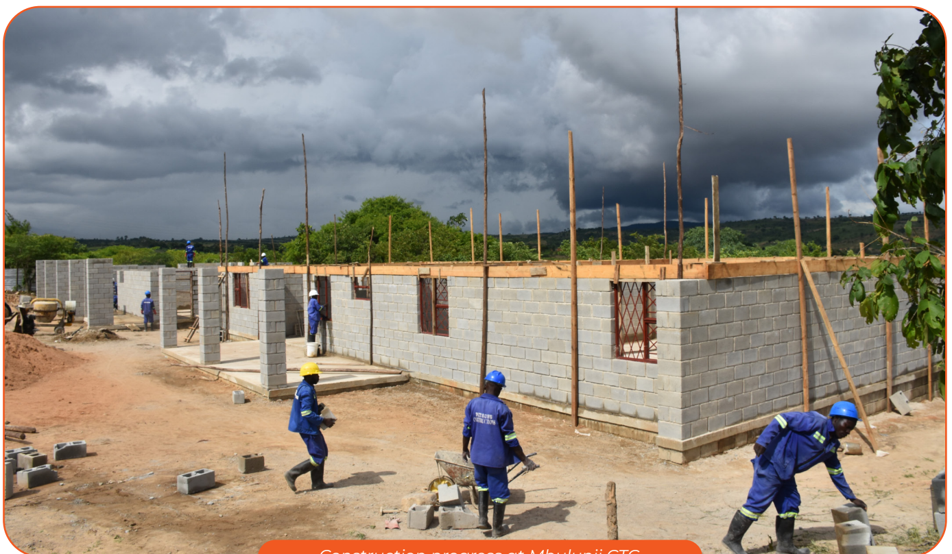
Construction progress at Mbulunji CTC
